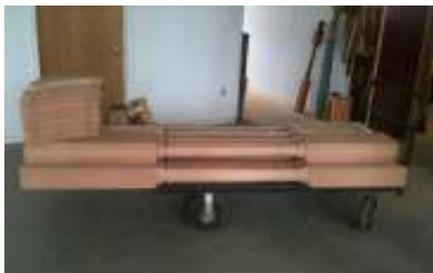
5 new porch posts and 5 repaired (rot cut off and new bottoms added). New are 5.44 x 5.44 x 102 inches in Spanish cedar.
